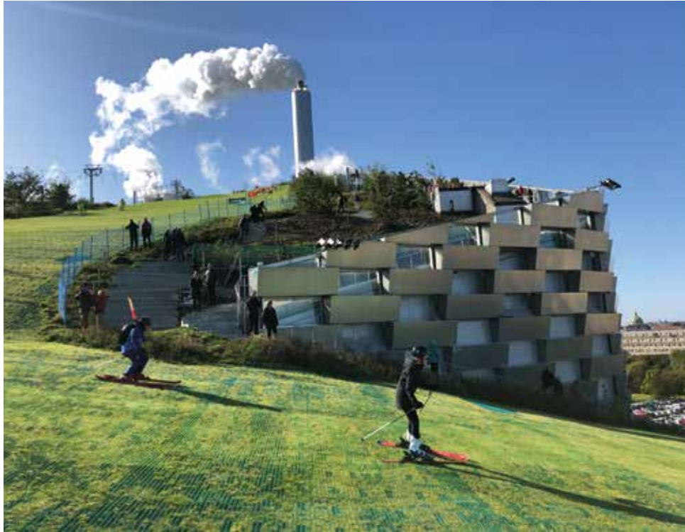
Incineration plant Amager Bakke, aka Copenhill, in the middle of the Danish capital: an artificial ski slope and recreational hiking area on top of a state-of-the-art waste-to-energy plant
